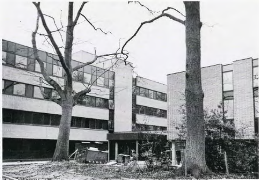
Office Block, Main Entrance and Conference Block, Shinfield Park.
